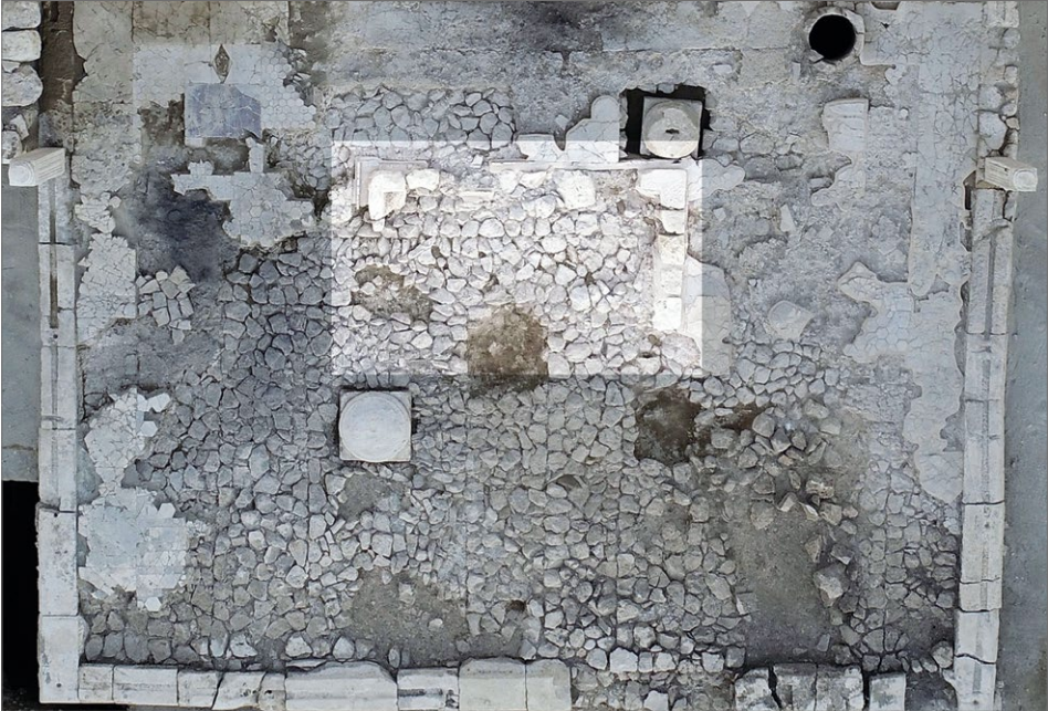
Fig. 11. Bema: altar, ciborium, templon stylobates and posts, sacred well and opus sectile (Photo C. Demirton)
