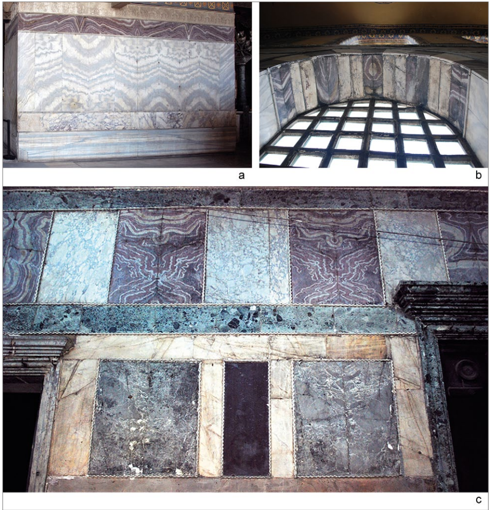
Fig. 8. Iasian marbles in Hagia Sophia: a – wall cladding in the galleries with the upper fascia made of red cipollino ; b – tiles in window archivolt of the galleries; c – book-matched panels in the endonarthex (Photos D. Peirano)
