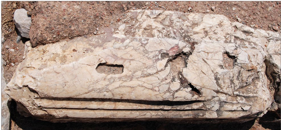
Fig. 11. Pavonazzetto block in the solea of the basilica of St. John in Ephesos (Photo D. Peirano)
