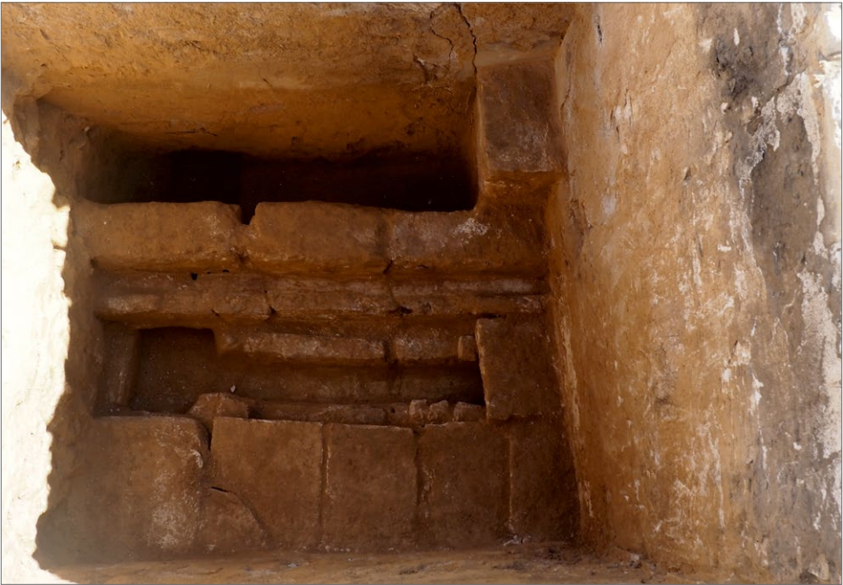
Fig. 5. Latrine in building H.39 (the bath facility is behind the wall on the right) (PCMA UW | photo O. Puzskarewicz)
