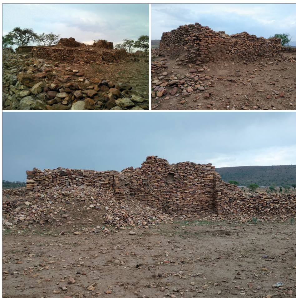
Fig. 7. Central building: top left, view from the northeast; top right, view of the western side from the northwest; bottom, detail of the southern side viewed from the southeast (Photos M. Gaudiello)
