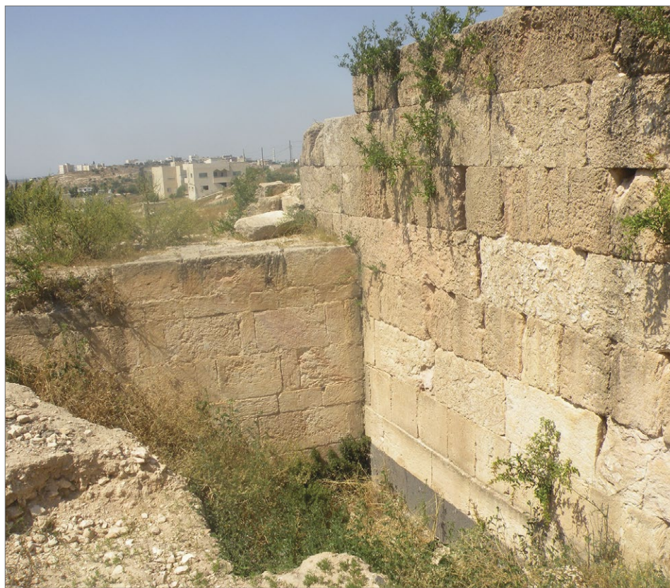
Fig. 16. The connection of the city wall section (on the left) with the theater wall (on the right) (Photo J. Młynarczyk, 2011)
