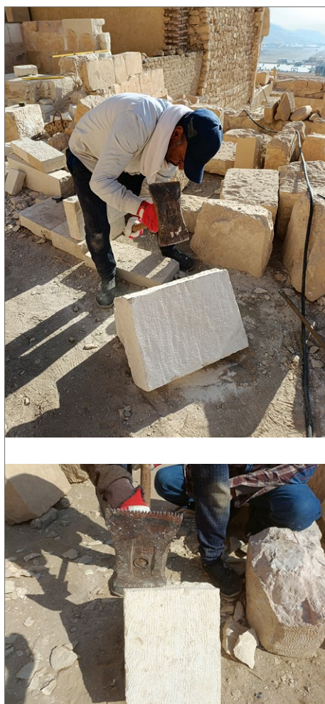
Fig. 6. Modern Egyptian toothed adze ( shahuta ), in use by stonecutter Sabr Ibrahim Hussein at Deir el-Bahari, 24.11.2024 (PCMA UW | photos D.F. Wiczorek)
