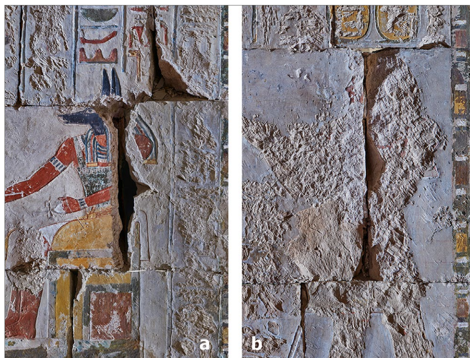
Fig. 10. Damaged walls during dismantling of the Niche: a) southern wall, b) northern wall. Damage on both walls was caused by prying the blocks apart with rods during the wall's disassembly. The marks show they were shifted sideways (to the left) using three rods simultaneously at the top, bottom, and middle. The central lever pressure caused severe damage to the blocks on the right side (PCMA UW | Photo M. Jawornicki)
