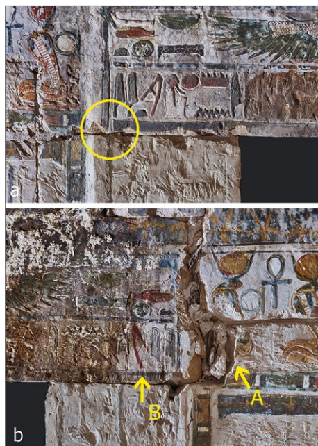
Fig. 14. a) Detail 1. Lintel of the portal in the western wall of the Sanctuary. Note, that the vertical strip does not align properly with the jamb. This part of the lintel preserves original decoration from the time of Hatshepsut. The cobra, the wing of the goddess, texts, and the bands are rendered consistently. The decoration differs on the opposite side of the portal (PCMA UW | photo M. Jawornicki, processing A. Kwaśnica); b) Detail 2. Right side of the portal lintel. The quality of the relief is markedly lower, as it was carved on a previously chipped surface. The most intriguing feature is the connection of the lintel block with the wall. To insert the lintel, a portion of decorated limestone blocks had to be cut out. A – filler material used to compensate for the mismatched edges between the lintel and wall, consisting of limestone rubble and mortar (no longer preserved). B – absence of the pet sign; text is only partially painted and lacks relief (Photo M. Jawornicki, graphic A. Kwaśnica)
