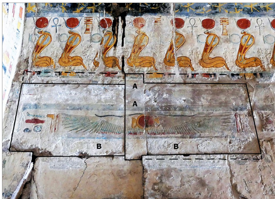
Fig. 18. Lintel of the portal leading to the Sanctuary. Two reused decorated blocks inserted into the wall. Dashed lines indicate the original block shapes. A – indicates pet stripes; two pet stripes with a gap between them form a decorative element not seen elsewhere in the temple. Originally, this must have been the lower level of the scene above. B – indicates remnants of hieroglyphic text added after the decoration above (Photo and graphic A. Kwaśnica)
