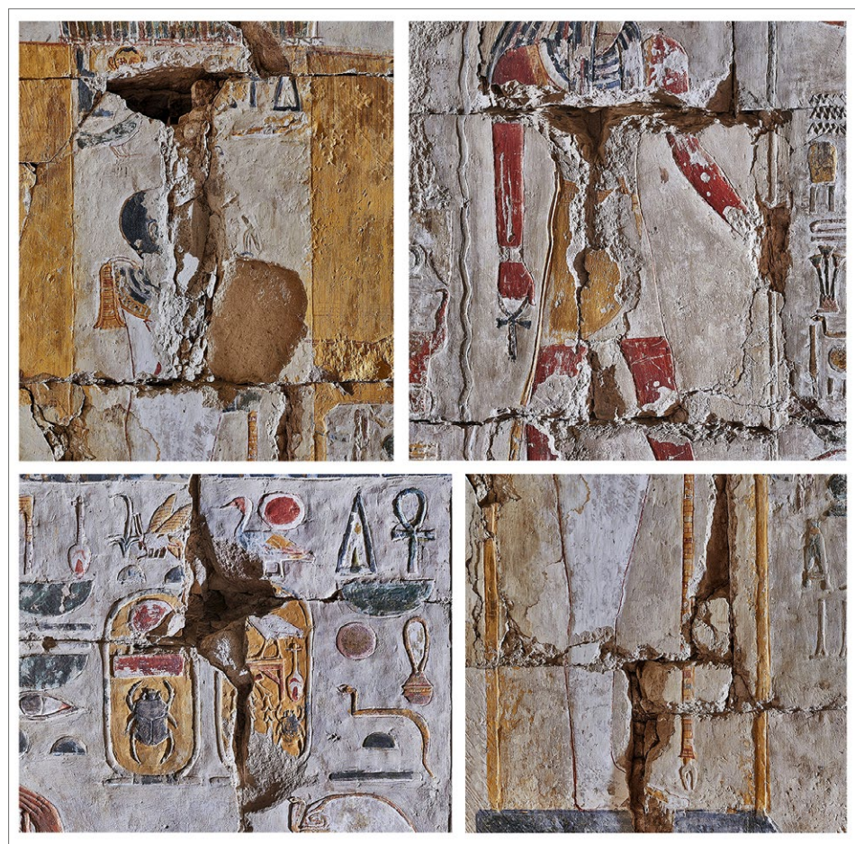
Fig. 5. Eastern wall of the Sanctuary. The large gaps between blocks are filled with crushed stone covered with polychrome plaster (PCMA UW | photo M. Jawornicki)
