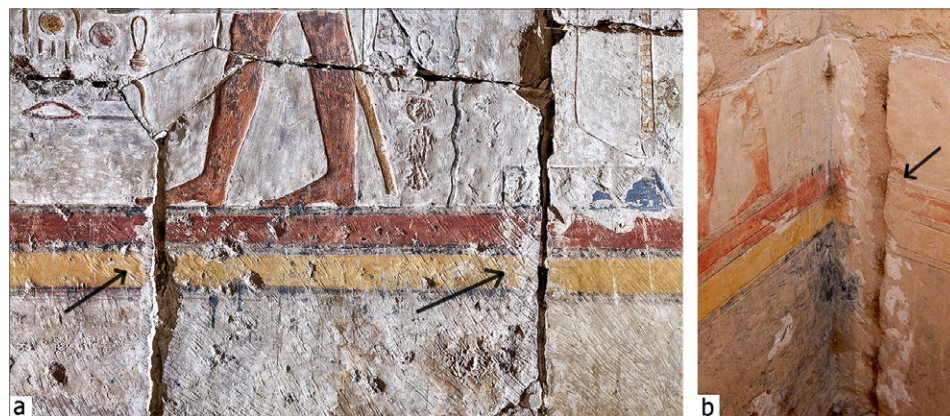
Fig. 12. The outer face of each block was shaved, including the decoration, to align the exterior surfaces of neighboring blocks after reassembly. This method was used in the Sanctuary (a) and in niches transferred to the Vestibule of the Chapel of Hatshepsut (b) (a: PCMA UW | photo M. Jawor-nicki; b: photo and processing A. Kwaśnica)
