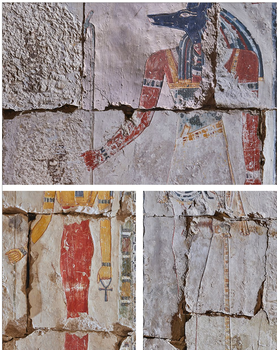
Fig. 8. Wall fragments of the Sanctuary. Marks show where rods (wedges) were inserted between blocks to pry them apart during dismantling. The rods acted as levers, damaging the edges of adjacent blocks (PCMA UW | photo M. Jawornicki)
