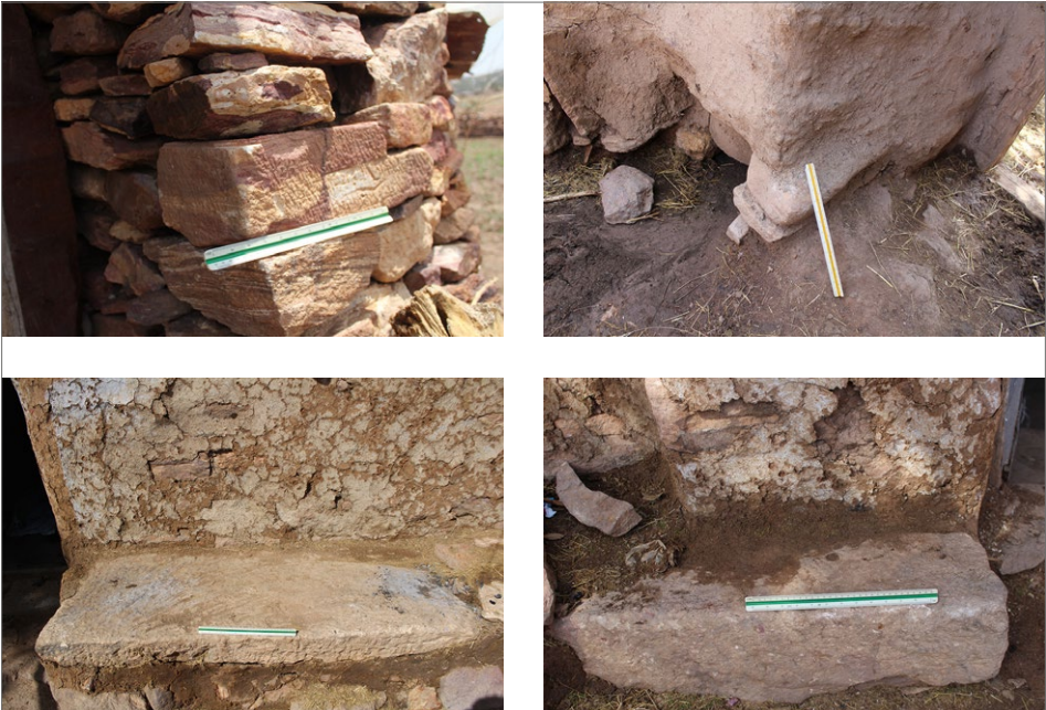
Fig. 3. Reused rectangular well-dressed stone slabs (Photos Mearg Abay Abebe)
