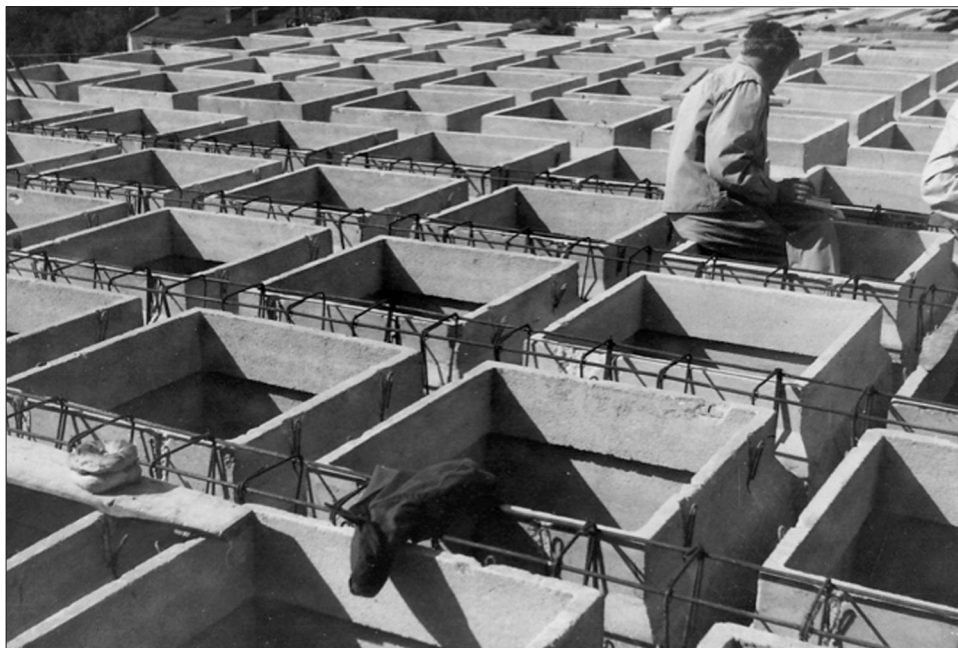
Fig. 12. Prefabricated coffers of the ceiling being joined with reinforced-concrete frames during the construction of the church of St. Michael the Archangel, 1960s, unknown photographer, Kinga Pieńkowska-Owsińska's archive
