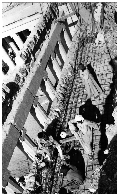
Fig. 10. Construction work installing the horizontal reinforced concrete slab at the back of the north wall of the Middle Terrace portico (Połozanin 1988: Fig. 8)
