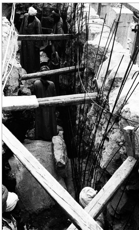
Fig. 9. Construction work behind the Northern Colonnade wall, installation of the reinforced concrete faceplate (Bielenia 1988: Fig. 5)
