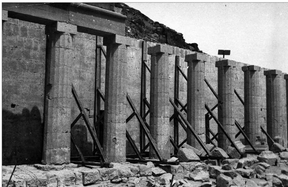
Fig. 7. Northern Colonnade, ad hoc timber scaffolding supporting the leaning wall (After Wysocki 1987: Fig. 9)
