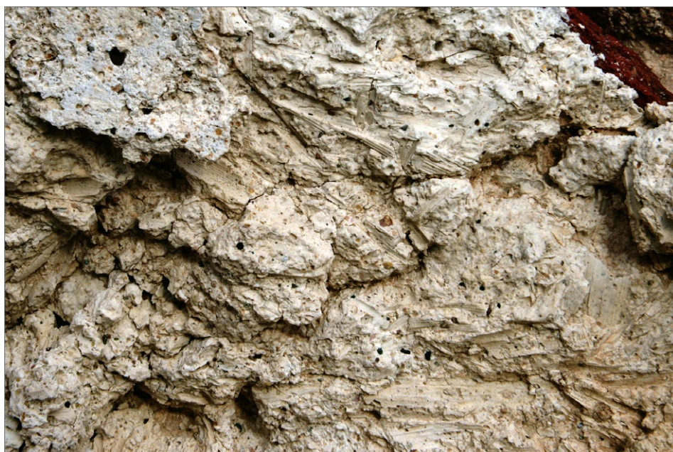
Fig. 16. Traces of organic fillers (fragments of straw) visible in the plaster on the eastern wall of room No. R.60 VT (Photo A. Tomkowska)
