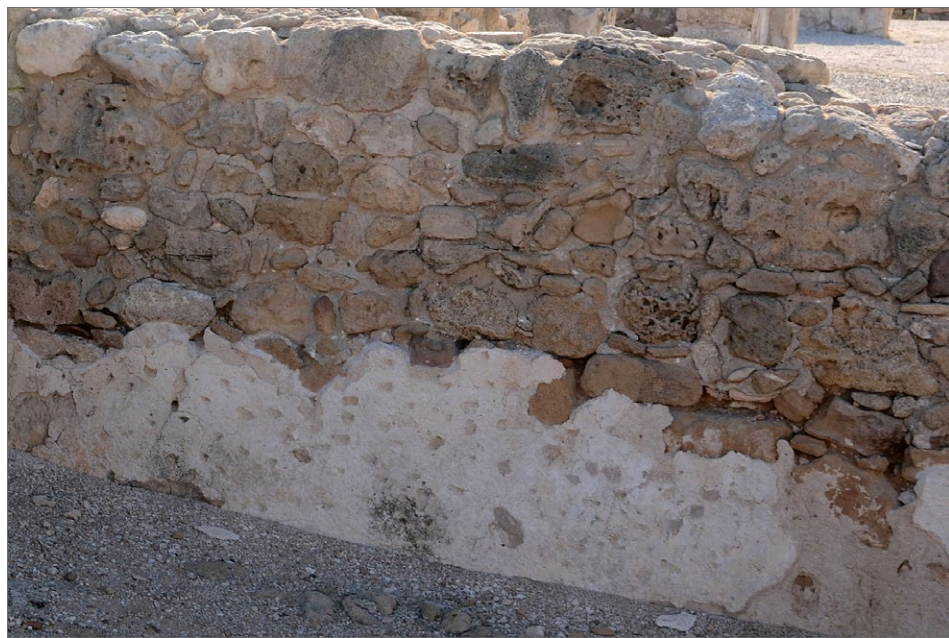
Fig. 25. Eastern wall of room No. R.42, showing clear signs of mortar keying on the plaster surface (Photo A. Tomkowska)
