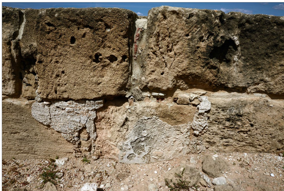
Fig. 15. Regular blocks of calcarenite used in constructing the apse of room No. R.39 VT (Photo A. Tomkowska)
