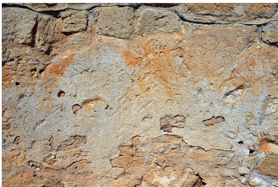
Fig. 17. Preparation of the base plaster for the upper layers: distinctive herringbone incisions on the western wall of room No. R.20 VT (Photo A. Tomkowska)
