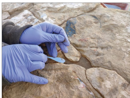
Fig. 9. Filling small cavities with a white cement-based mineral mortar (PCMA UW | photo K. Prus)
