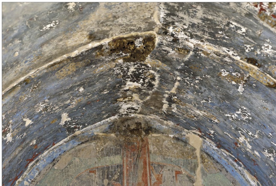
Fig. 8. Vaulted ceiling in a poor state of preservation, with visible remains of wasp nests, as well as bird and bat excrements (PCMA UW | photo P. Staszkievicz)
