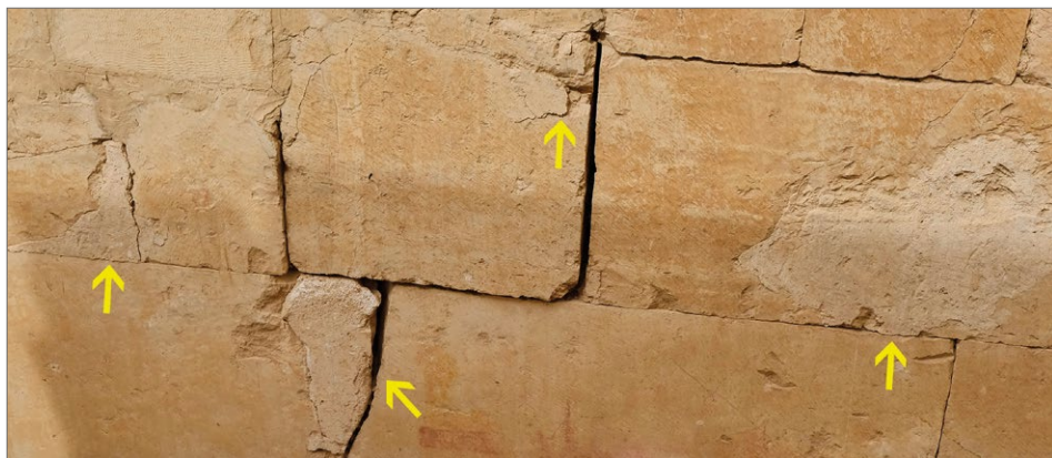
Fig. 25. Eastern wall of Niche B in the Room with a Window. Arrows indicate cavities patched with lime mortar most likely at the time of erecting the niches (Photo M. Jawornicki; processing A. Kwaśnica)
