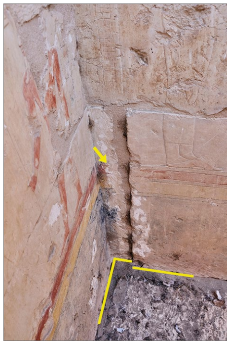
Fig. 24. Southwestern corner of Niche B. The faces of adjacent blocks do not form a single plane. In the time of Hatshepsut, both blocks were cut, plastered and covered with polychromy. Traces of ancient plaster are still visible on the surface (Photo M. Jawornicki, processing A. Kwaśnica)
