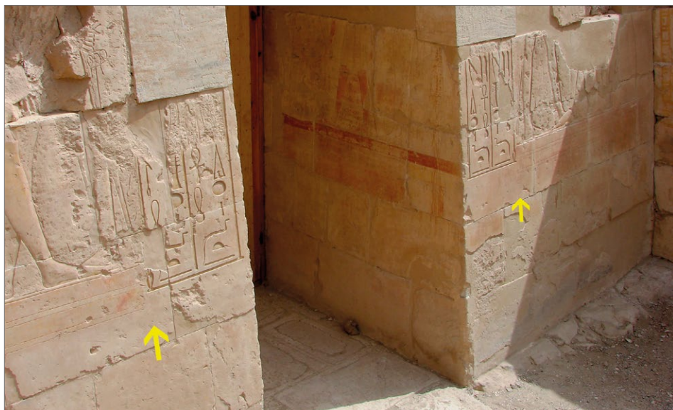
Fig. 5. Portal lacking a band around the entrance. Arrows indicate the place where it should have been. Decorations were executed on a flat wall, originally meant to be plain [see Fig. 3:4] (Photo and processing A. Kwaśnica)
