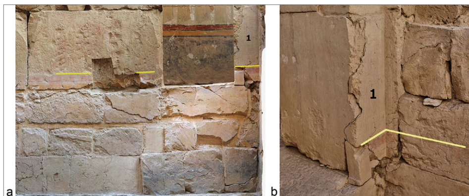
Fig. 20. Connection of the eastern and southern walls of the Vestibule of the Chapel of Hatshepsut: a – the dado rail on the eastern wall of the vestibule (PCMA UW | photo M. Caban, processing A. Kwaśnica); b – the dado rail on both walls is on the same level (Photo M. Jawornicki, processing A. Kwaśnica)
