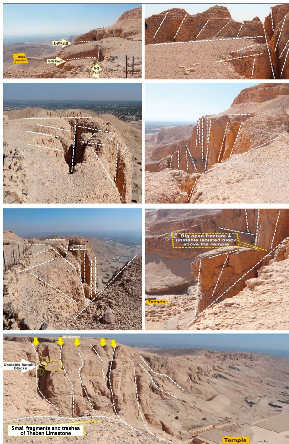
Fig. 7. Intersections between E-W and N25°E faults, causing hanging blocks, big open fractures and unstable isolated blocks above the Temple (© Authors)
