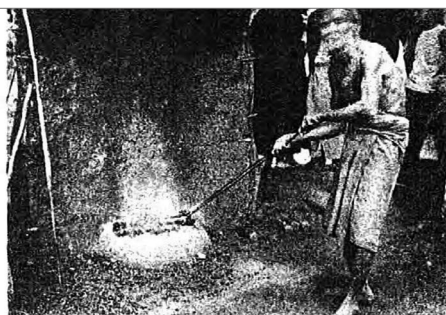
Steel furnace; removing crucibles.
