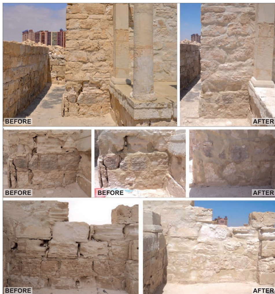
Fig. 8B. Commemorative monument before and after completion of work in the 2018 season: details of the wall, view from the the north and south (Polish–Egyptian Conservation Mission | photos W. Grzegorek)
