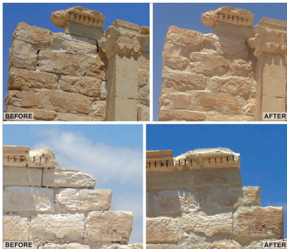
Fig. 8A. Commemorative monument before and after completion of work in the 2018 season: details of the wall (Polish–Egyptian Conservation Mission | photos W. Grzegorek)
