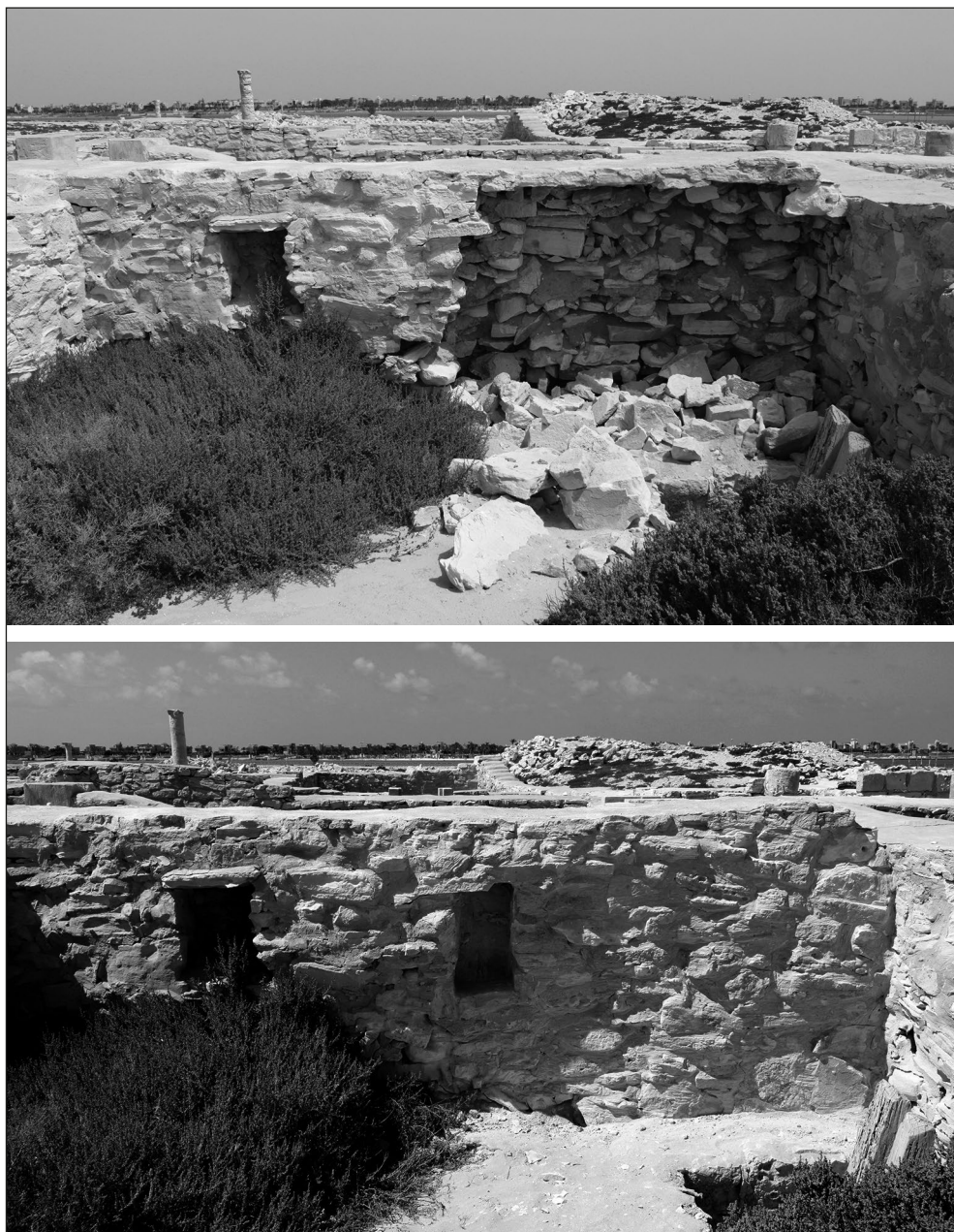
Fig. 10. Conservation maintenance in House H9: top, a wall in collapsed condition after the winter rains; bottom, after reconstruction in 2016 (PCMA Marina el-Alamein Conservation Mission/photos R. Czerner)
