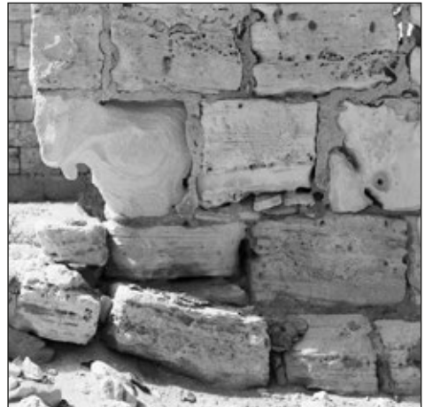
Fig. 11. House H21N: losses of stone blocks in the wall next to the passages (PCMA Marina el-Alamein Conservation Mission/photo P. Zambrzycki)
